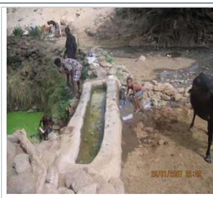
Figure 5. Rehabilitated livestock watering trough in Elebaha Kebele
